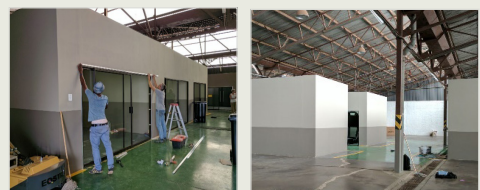
Construction is underway at MCC's new eXtract Operator Training Academy.
